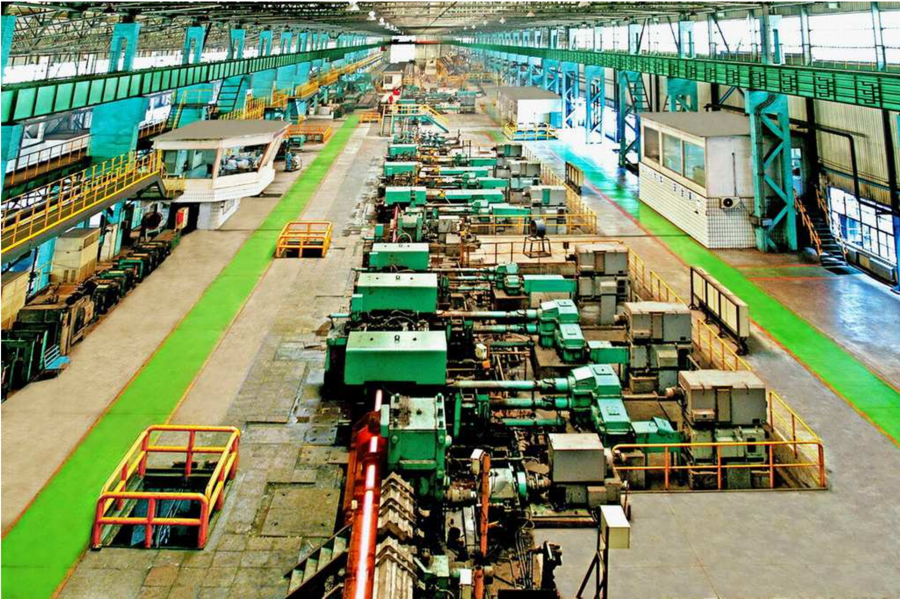
Bar and wire rod rolling mill:H-V×20stand+Block×10stand/SMS (Dalian)
